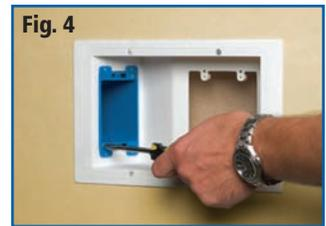
1. Locate studs and determine if they are 16" or 24" apart. If 16" apart, measure a maximum of 3" from edge of stud to determine plate location. If 24" apart, center plate between studs. Note: Low voltage side must be 3" from stud.
